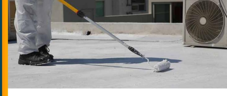
Elastomeric Water Proof Liquid Membrane
